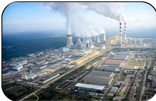
Belchatow power plant 5000 MW , Poland
