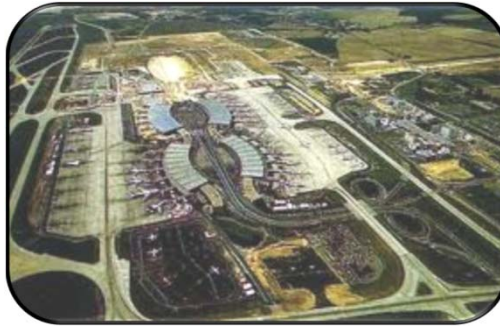
Liaison Interne Satellite Aéroport – Internal Airport Station Satellite Link
