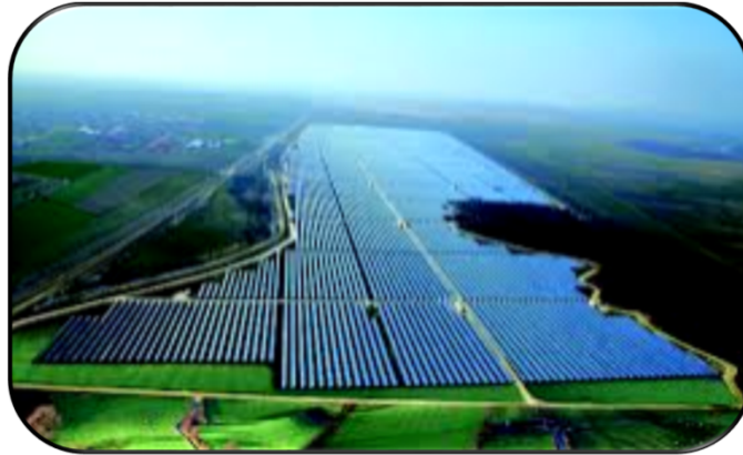
Karazdalovo solar power plant 60MW , Bulgaria
